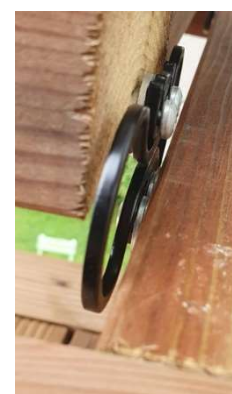
Picture 3B: Space for the spring and washers is 7 mm at both ends, 14 mm in total
