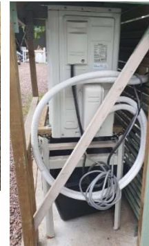
Picture 8. Outdoor unit heavier end and 360-degree bend to allow flexibility
