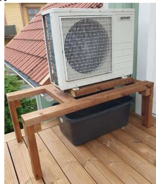
Picture 10. Finalized floor stand from above (Longitudinal beams are longer in the picture 140 cm vs instructed 100 cm)
