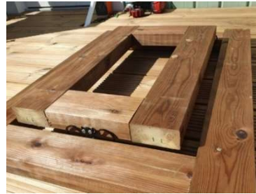
Picture 7. Upper frame installed on top the isolators
