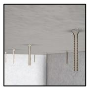
Install the acoustic hanger lower parts inside the GK60 ceiling profile. All acoustic hangers can be installed inside the GK60 ceiling profile before connecting the acoustic hangers to the Nonius upper parts.
