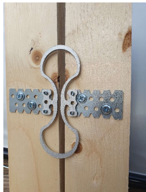
AWT128NN between two laminated veneer lumber beams, total width 128 mm
